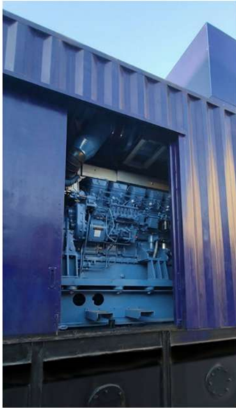
MGS2500R's S16R2-PTA Engine, the legendary powerhouse
