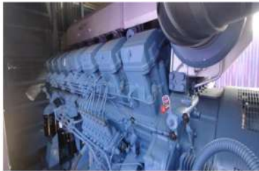
MGS2500R's S16R2-PTA Engines
